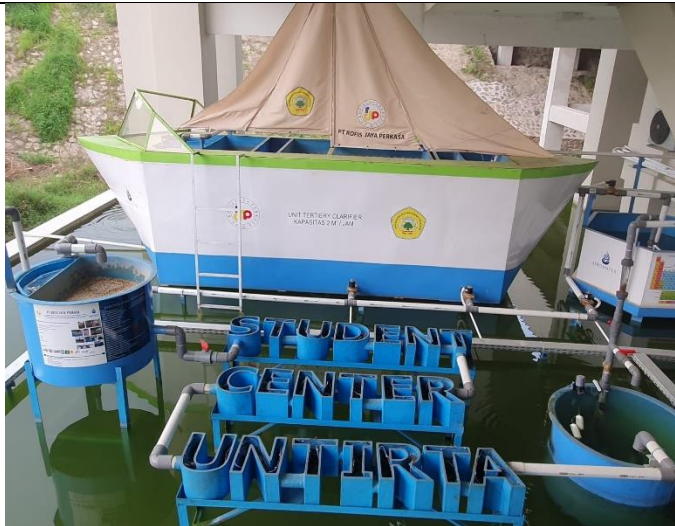
Wastewater and rainwater treatment equipment using Electro System
