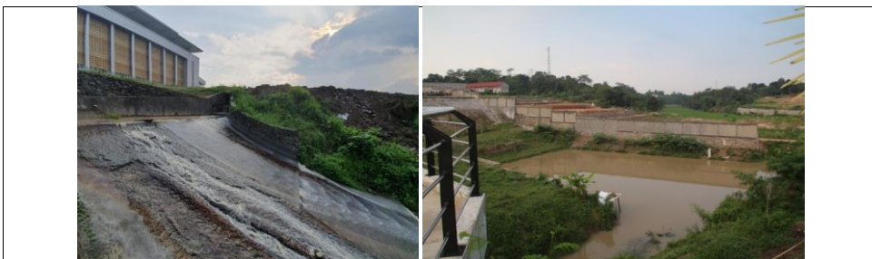
Figure 4.6 Retention Pool as flood control and water management at Untirta Sindangsari campus
